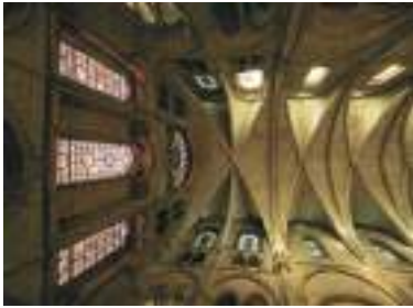
Picture 24 – Cross vaulting from the end of the 12th century – photo TD
