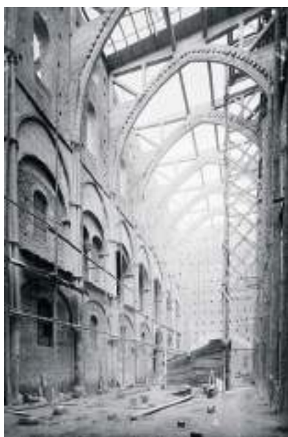
Picture 36 – Reconstruction of the nave (1920s) © Ministry of Culture - Médiathèque de l'architecture du patrimoine (diffusion RMN)
